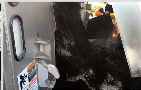
Asphalt can be unloaded incrementally into the paver.
